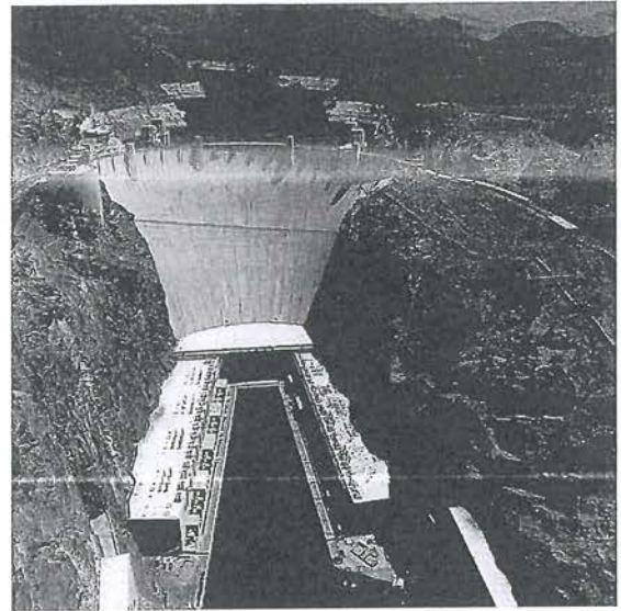
A large hydroelectric plant at the base of Hoover Dam on the Nevada/Arizona border.
